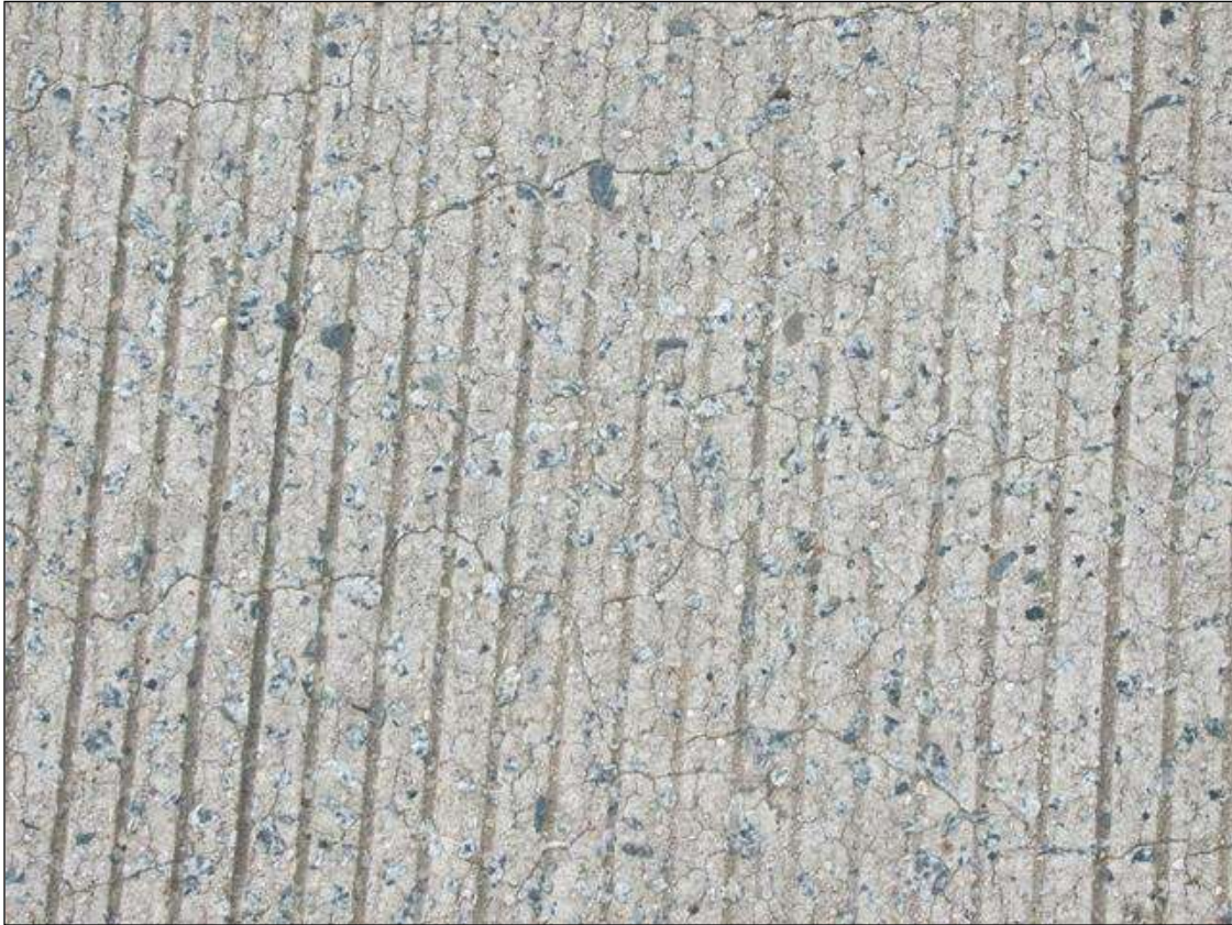
HL. MAP CRACKS IN ALL SPANS
