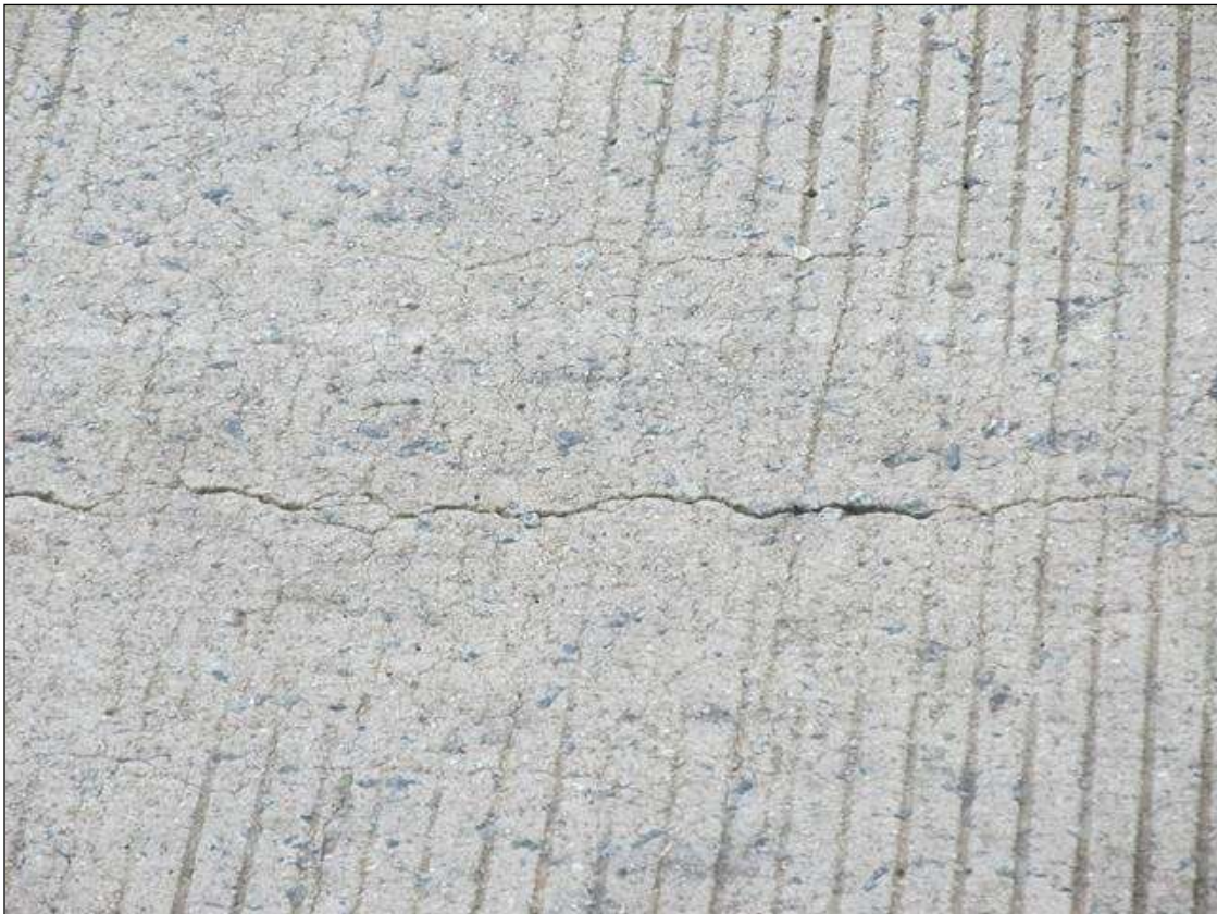
HL. TO 1/16" WIDE LONGT. CRACKS IN BOTH APPROACH SLABS
