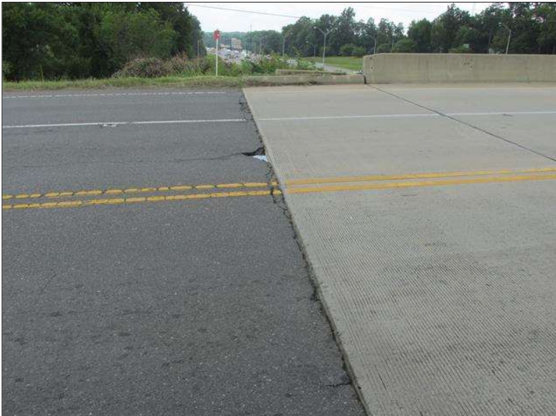
BOTH APPROACH ROADWAYS HAVE POTHOLES UP TO 3" DEEP X 1 FT. IN DIA. AND ARE CRACKED AND BREAKING UP AT THE APPROACH SLAB
