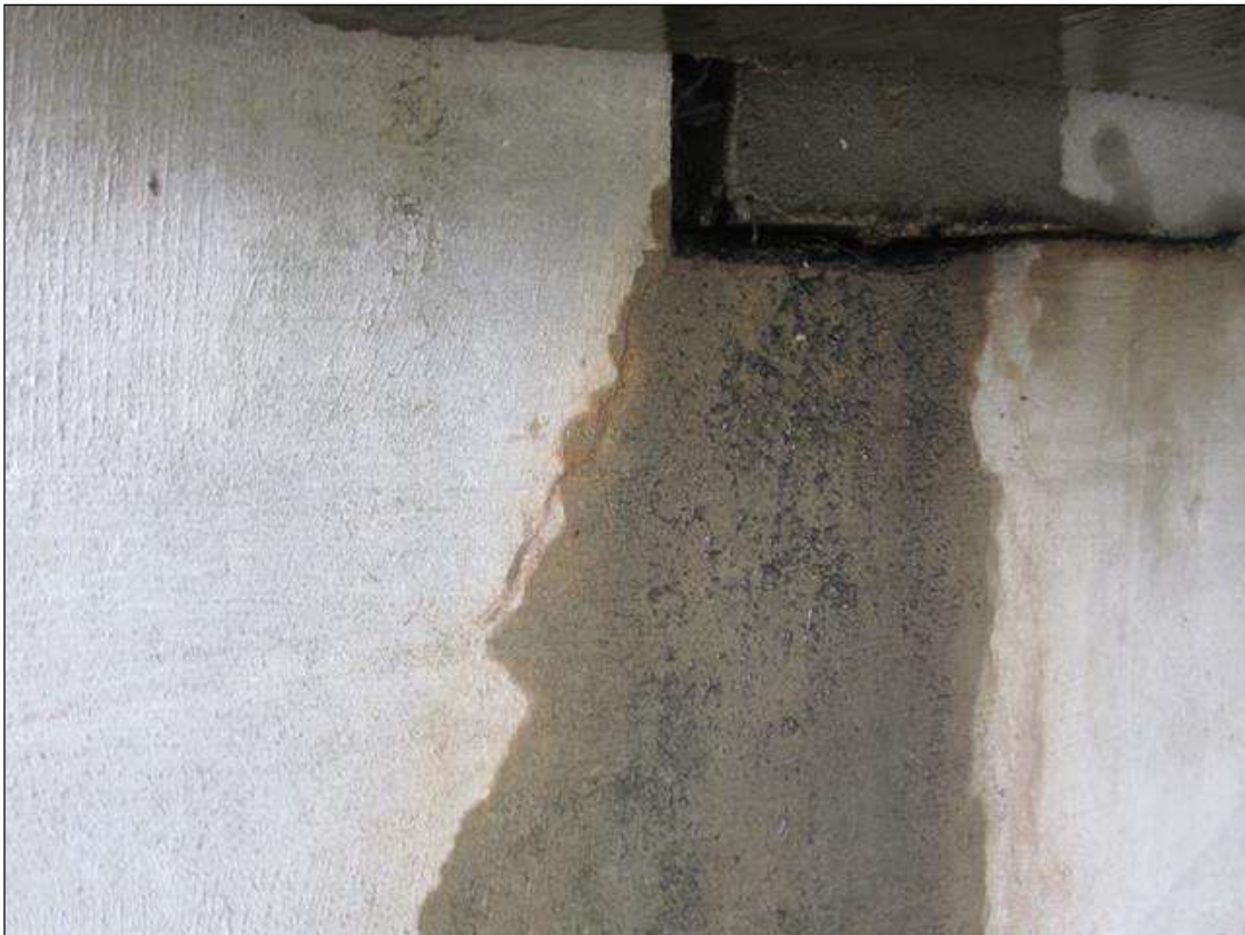
HL. DIAGONAL CRACKS IN BOTH ABUTMENT BACKWALLS
