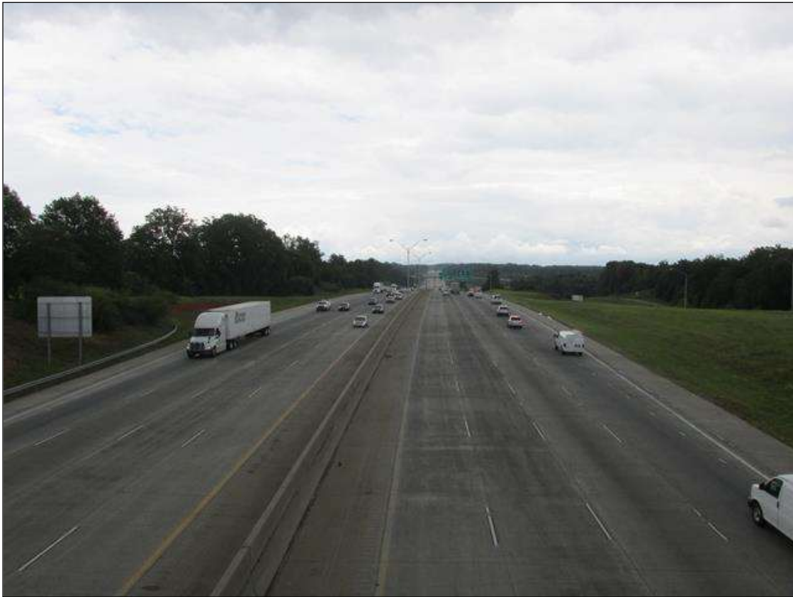
RAMPS LOOKING EAST
