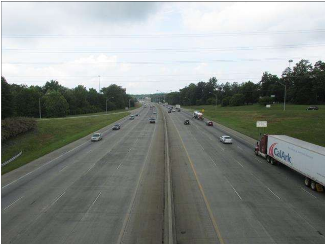
RAMPS LOOKING WEST
