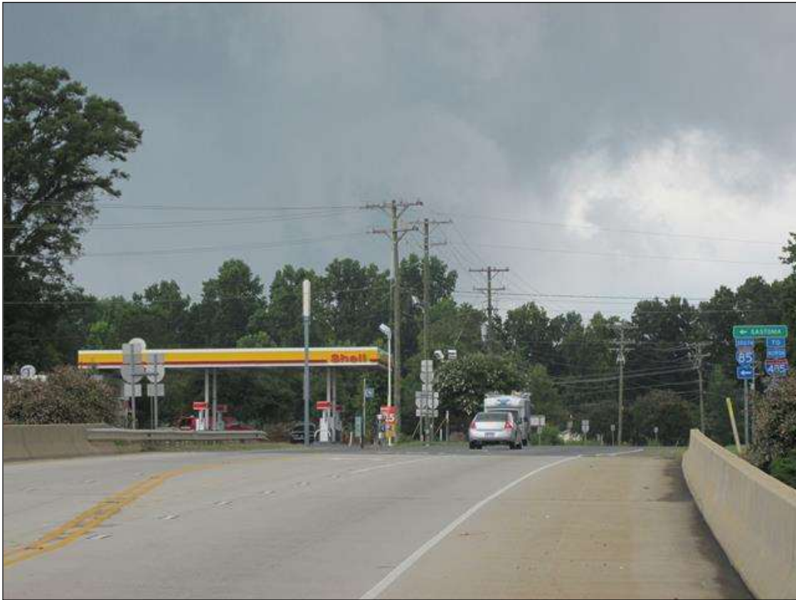
GUARD RAIL LOOKING NORTH RAMP LOOKING NORTH
