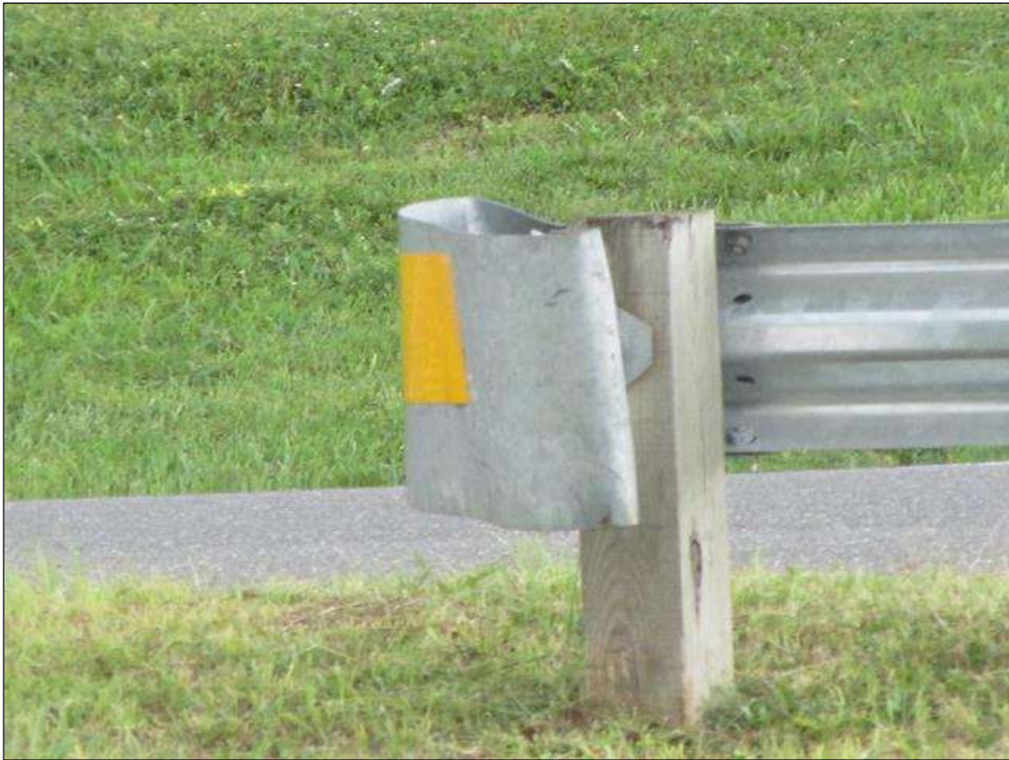
GUARD RAIL TERMINAL END AT THE NW END NE AND SE SIMILAR
