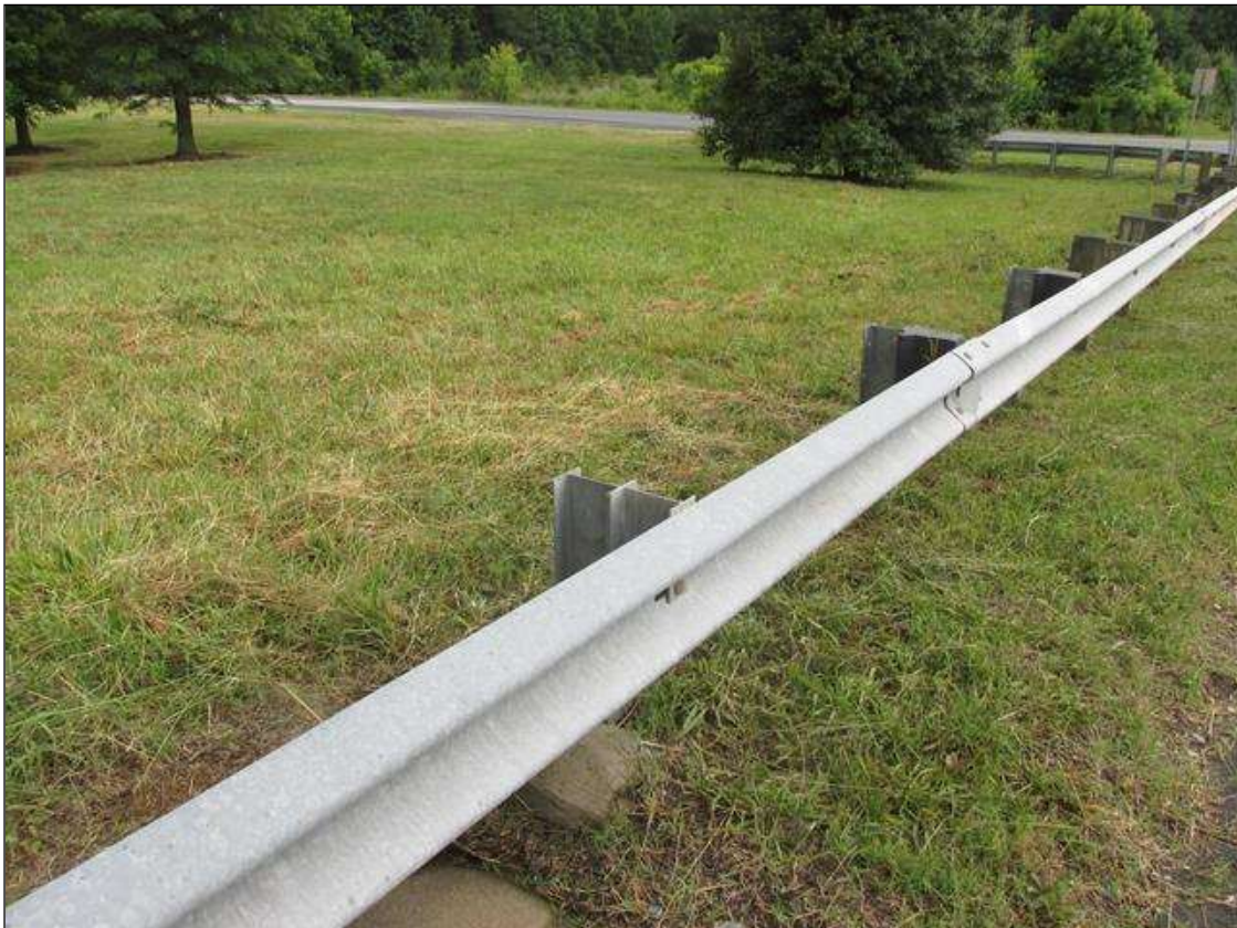
GUARD RAIL POST SPACING IN THE MIDDLE
