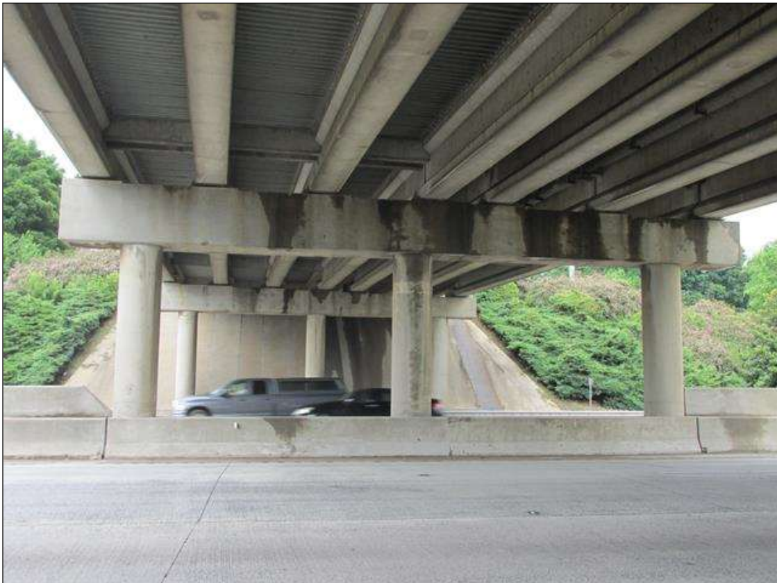
PIER 1 LOOKING NORTH
