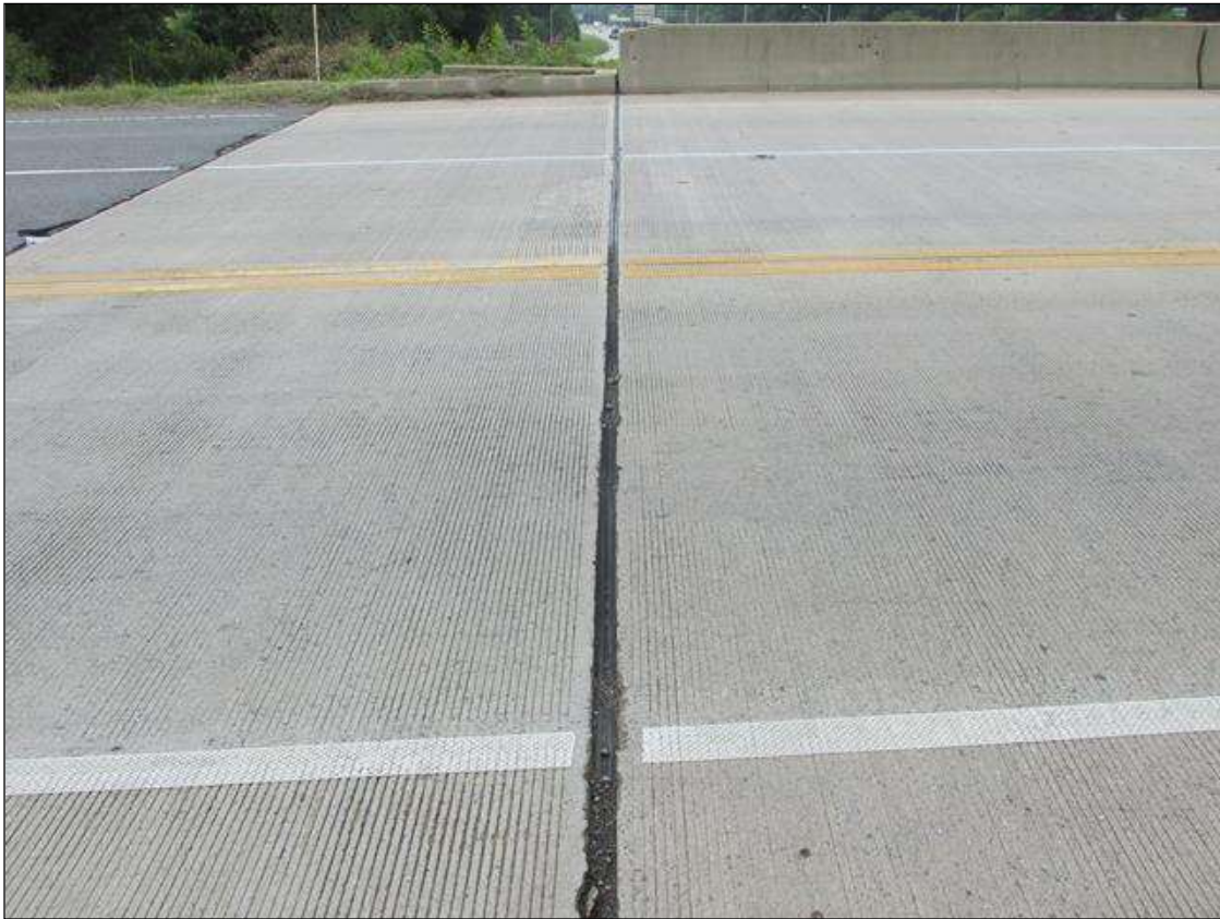
EXPANSION JOINTS AT THE ABUTMENTS AND PIERS
