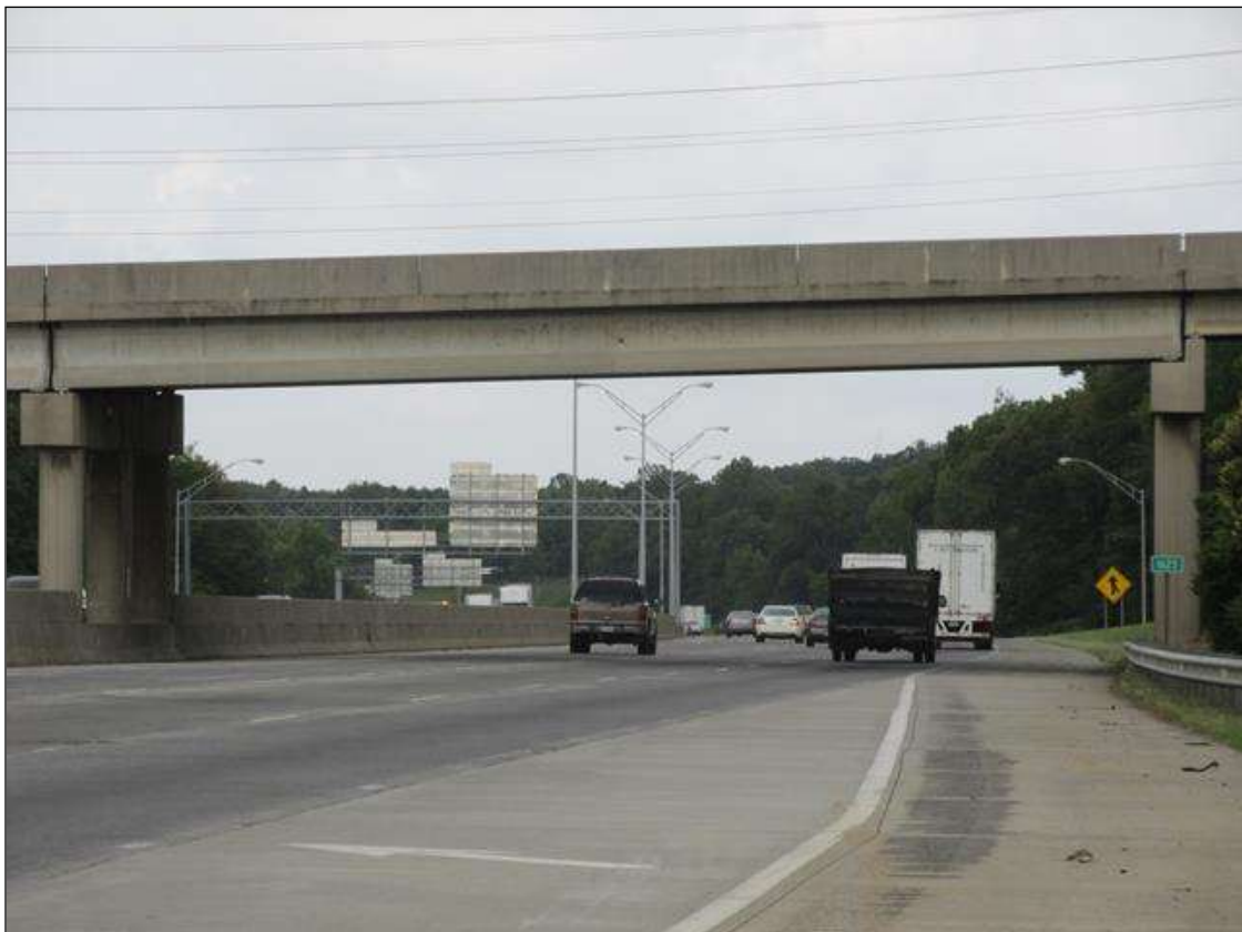
WEST OPENING, SPAN 3
