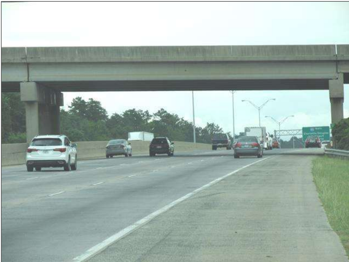
EAST OPENING, SPAN 2
