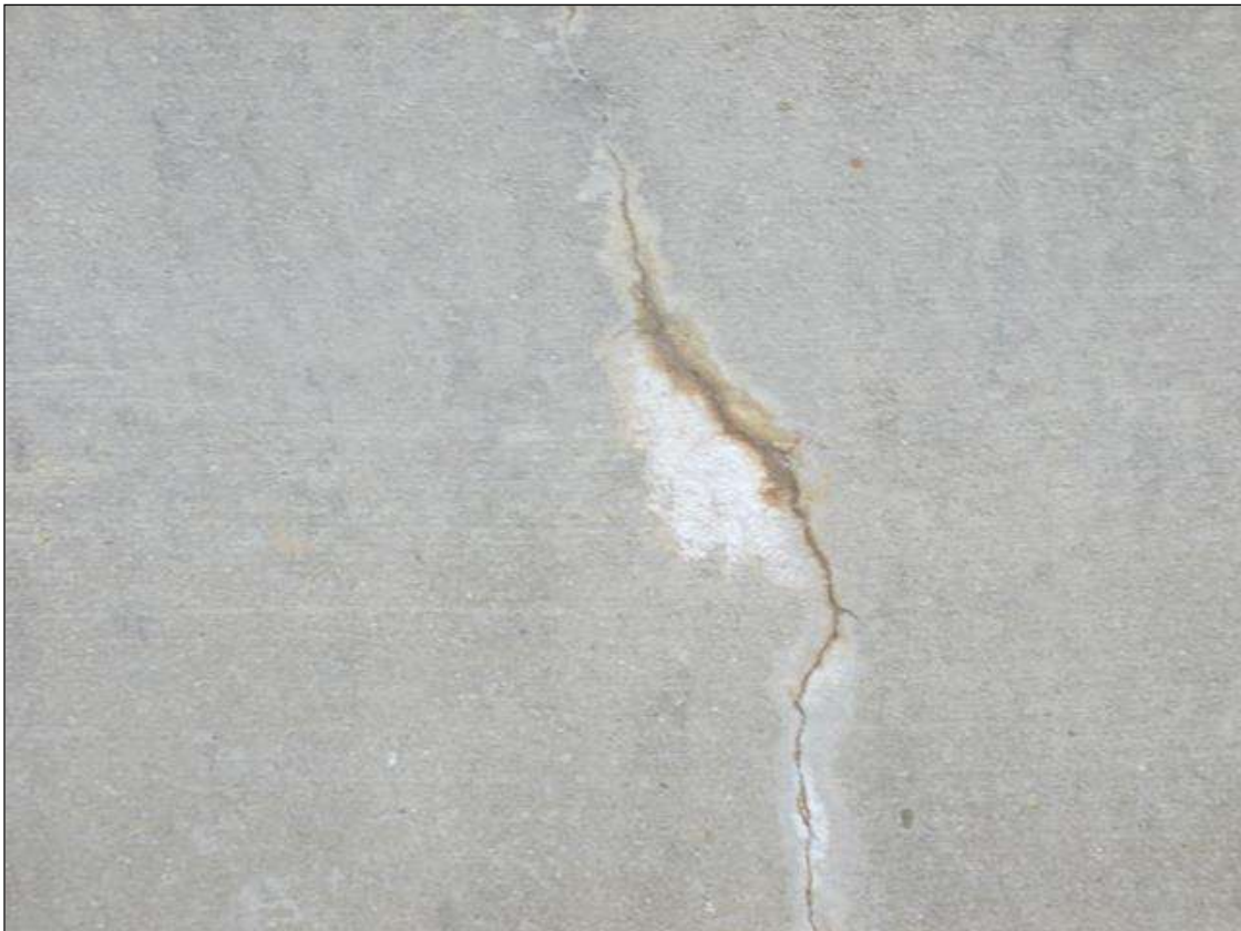
HL. VERTICAL CRACKS IN BOTH RAILS
