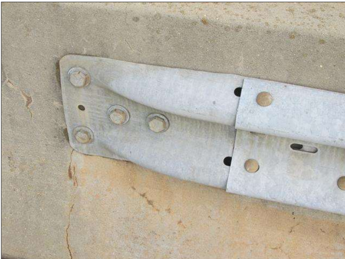
GUARD RAIL CONNECTION SE CORNER NE AND NW SIMILAR
