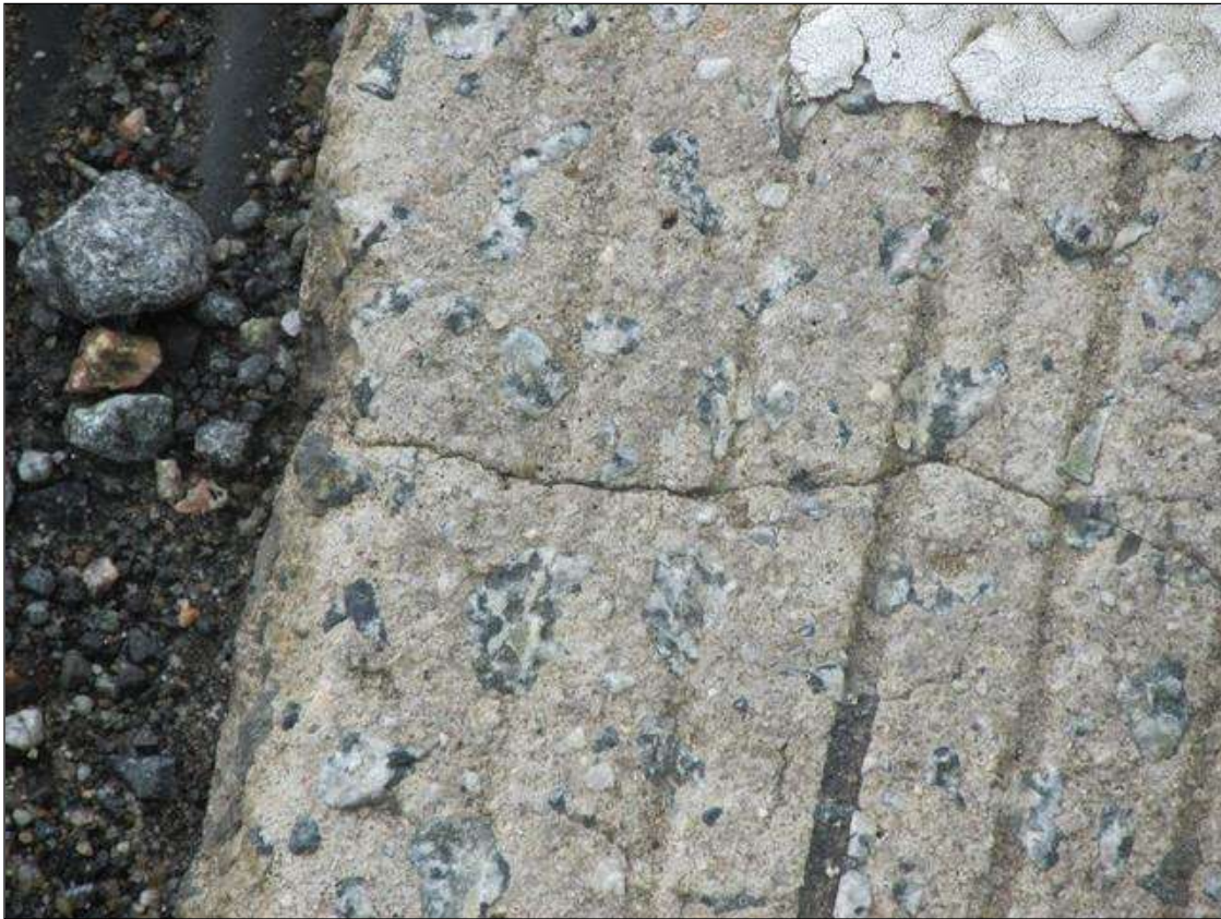
HL. LONGT. CRACKS IN THE SPAN ENDS
