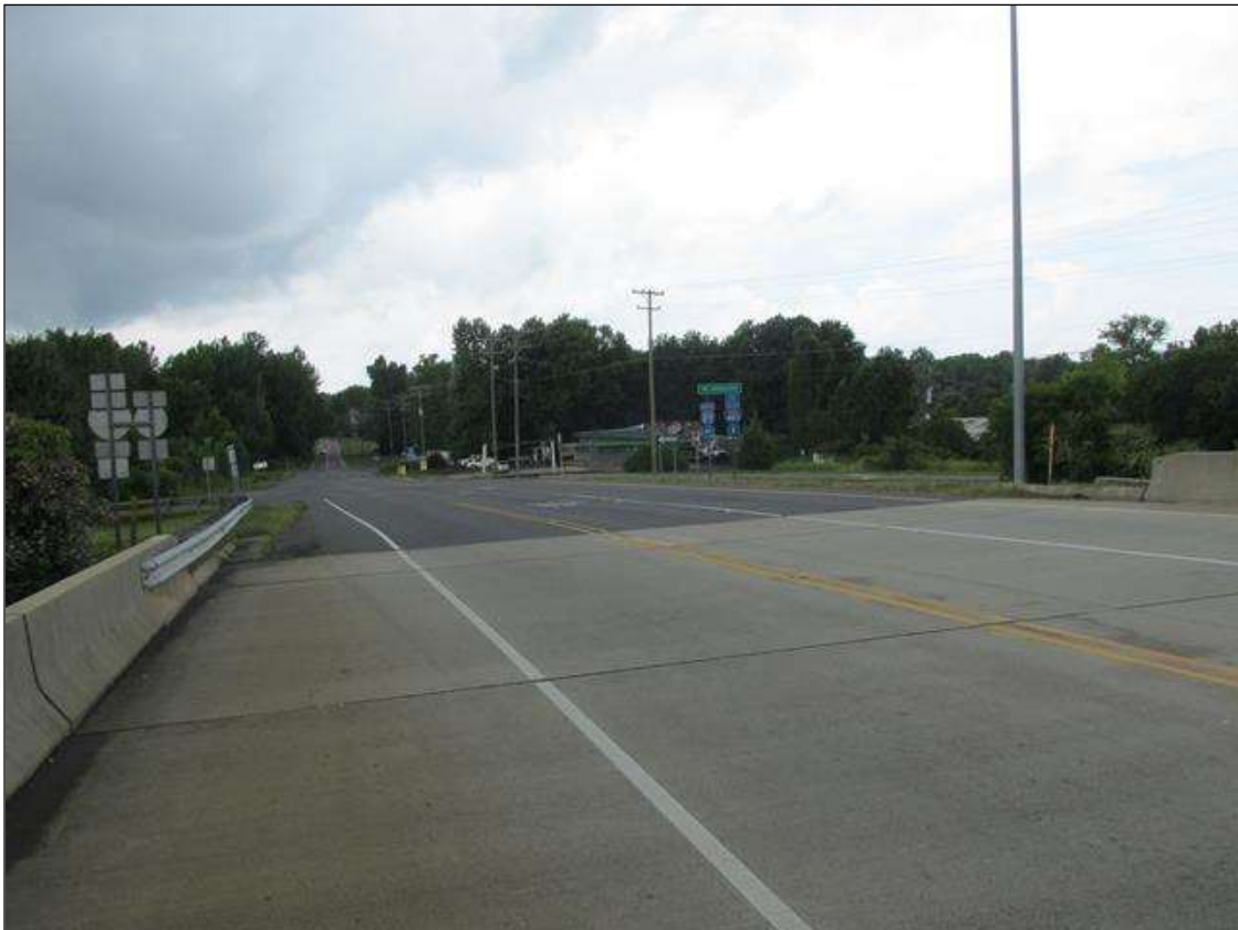
GUARD RAIL LOOKING SOUTH RAMP'S LOOKING SOUTH
