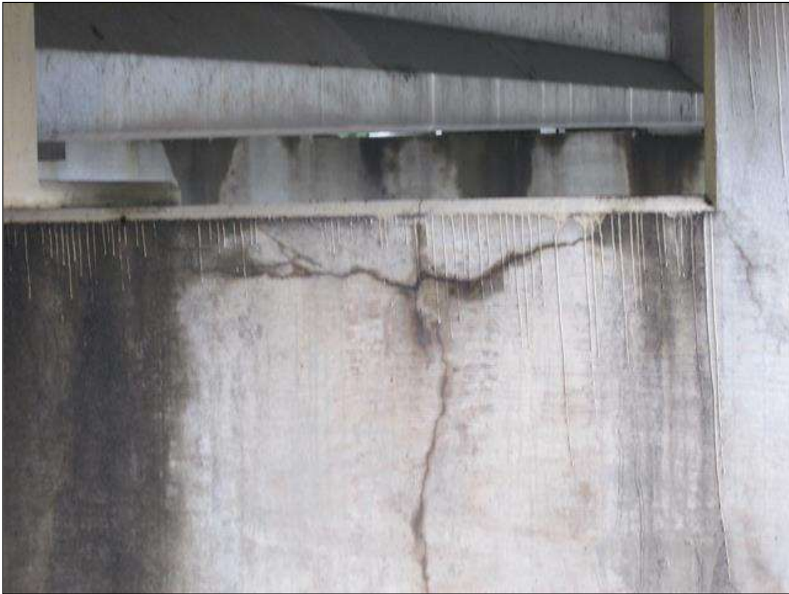
CRACKS IN THE SOUTH FACE OF PIER 1 CAP OVER COLUMN 3 UP TO 1/16" WIDE
