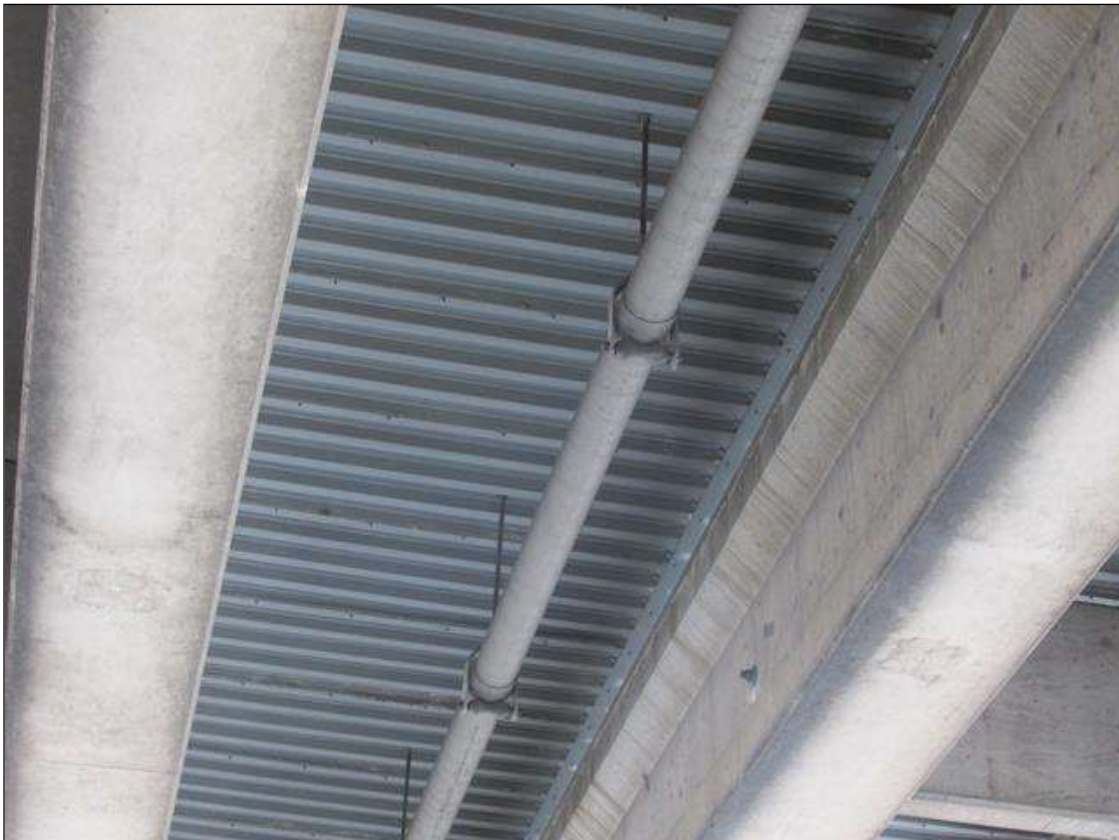
1 - 8" UTILITY IN BAY 5
