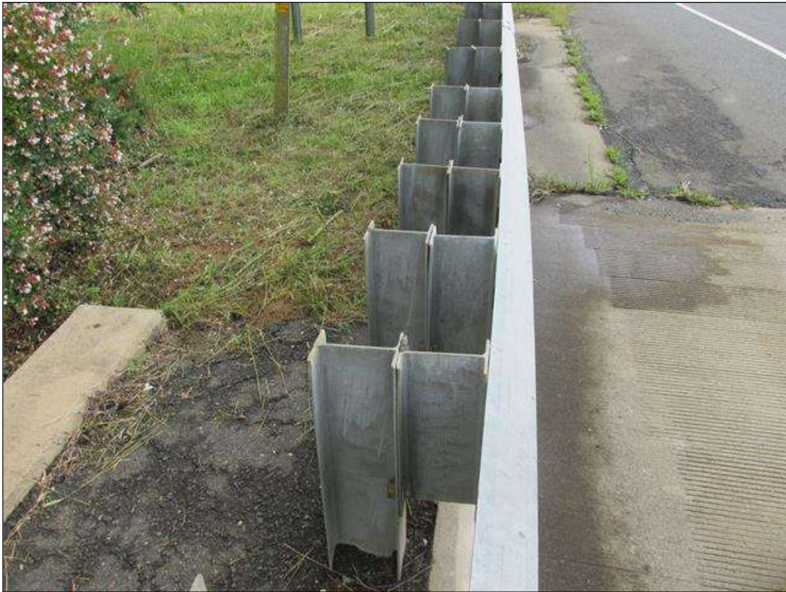
GUARD RAIL POST SPACING AT THE SE CORNER NE AND NW SIMILAR
