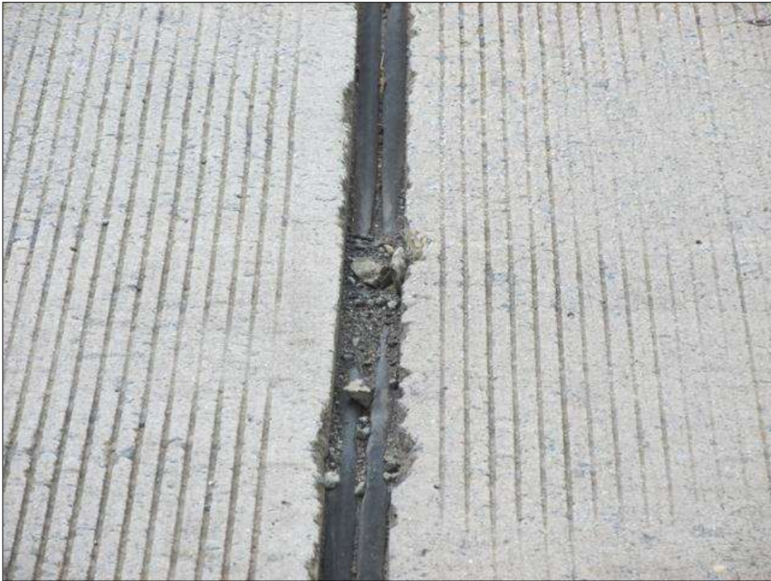
ALL EXPANSION JOINTS ARE SETTLED AND LEAKING
