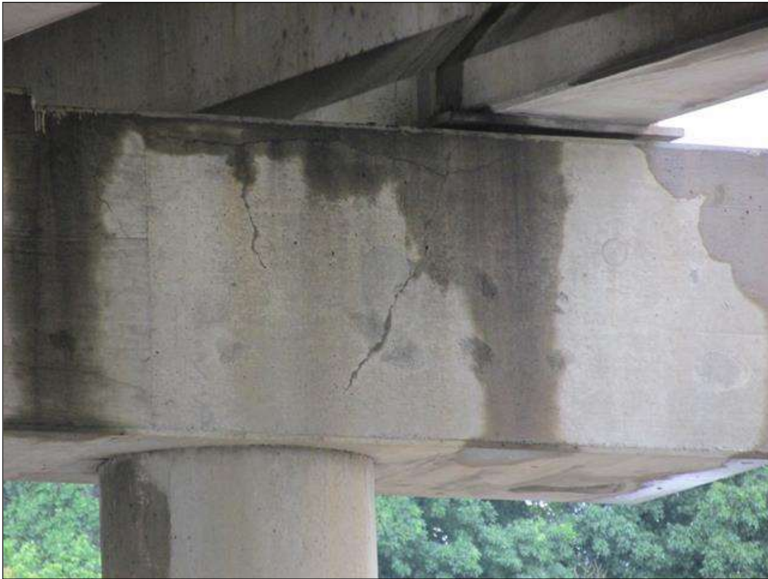
HL. DIAGONAL CRACKS IN THE SOUTH FACE OF PIER 2 CAP ABOVE COLUMN 3
